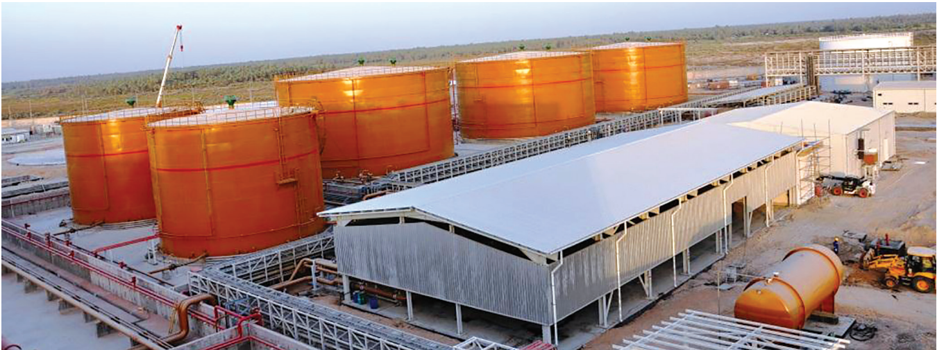
Nainawa Power Plant - Irak
