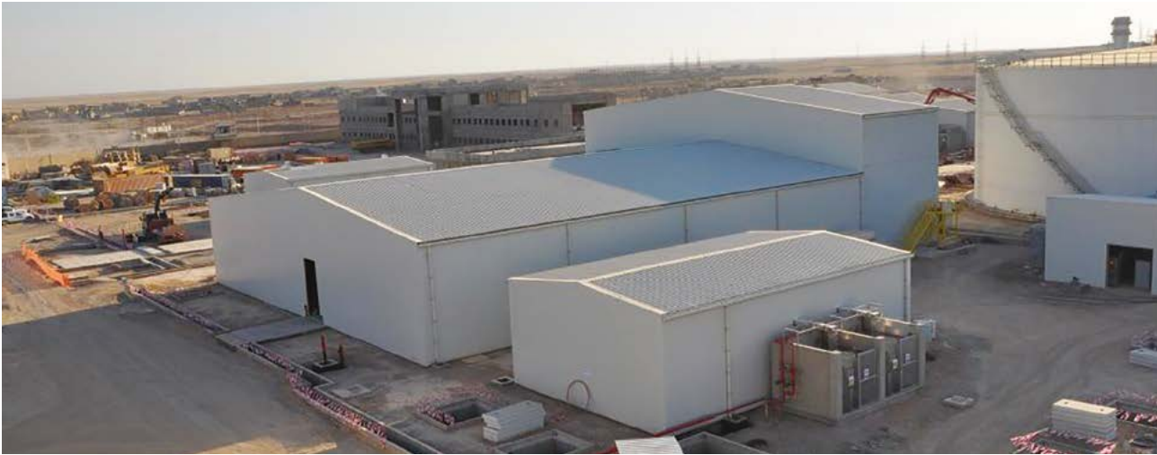
Al Kharirat Power Plant - Irak
